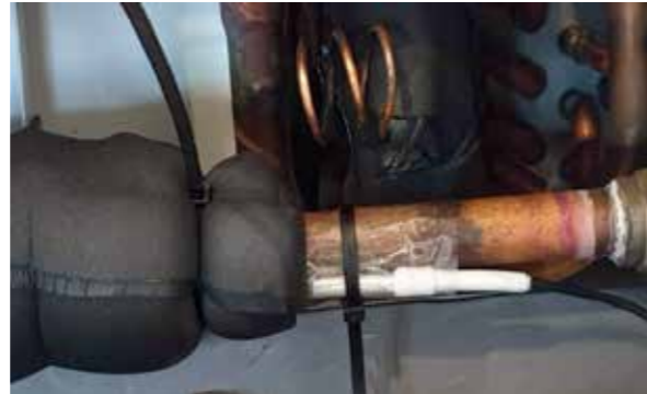
Place sensor on copper pipe
