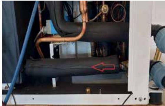
Move isolation back as far as possible
